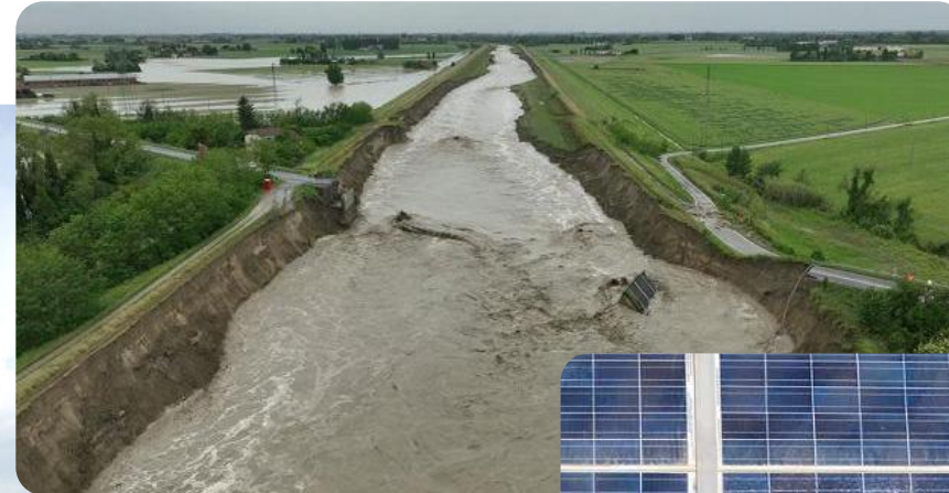
Bridge failure due to flood, May 2023 (Molinella di Budrio, BO) ( rainews.it )
